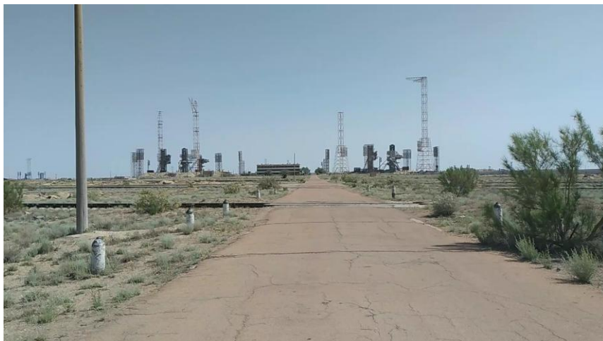
Launch complex "N-1", MTKS "Energia-Buran"
